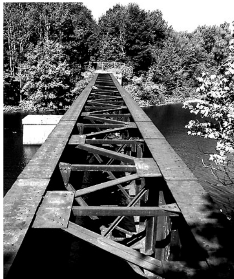
Future trail bridge near Blackstone, MA
